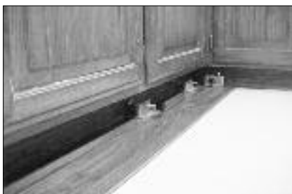
Job layout and determining an appropriate starting point is also very important with glueless laminate installations. The installation should be “balanced” with nearly equal panel widths at the sides and no panels shorter than 12" at the length walls. Sometimes it is advantageous to start the installation in areas that would be difficult to tilt in the last row, for example under cabinets, door casings, etc.
