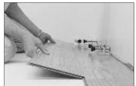
Begin second row with at least 12" stagger of end joints, assemble the first panel in the second row to the adjacent panel in the first row by slightly angling tongue into groove until plank locks into position. Insert the tongue at about a 20° angle and lock the planks together. (Use non-marring blue tape to secure the panel across the assembled joint to hold it in place.)
